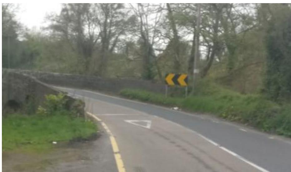
*Example of a Give-Way Shuttle at a Pinch-Point (N66 near Kilcreest, Co. Galway)*
