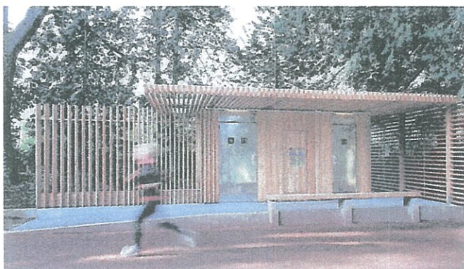
Example Pic 1; Small WC block in forest
