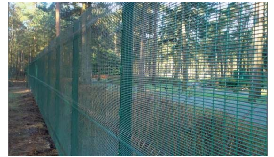
Powder Coated Green Paladin type fencing to secure with neighbouring residences where necessary. To be planted in association with dense shrubs/ hedgerows
