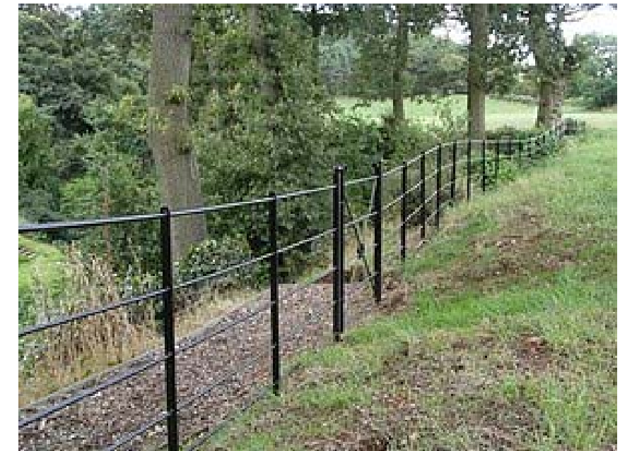
Estate type railings where required along steep banks of Glendoo river or to discourage access to habitat zones
