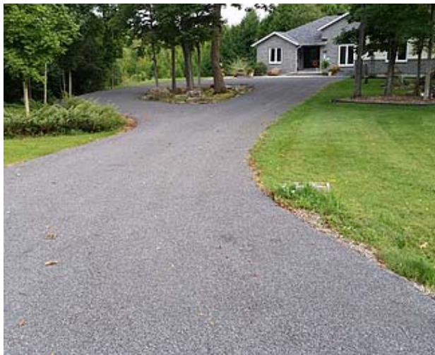
Where asphalt roads required in access areas / drives – finish to be select applied aggregate to ensure a rural character retained
