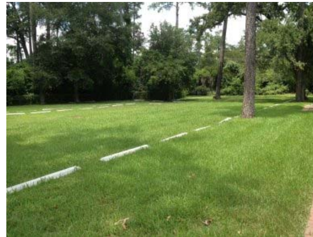
Permeable green reinforced grass areas for parking
