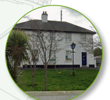
4. Rathcoole Garda Station
