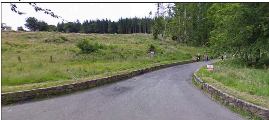
Figure 12.56 The boundary wall to the Coillte lands at Montpelier hill is by contrast a low 20 th century wall
