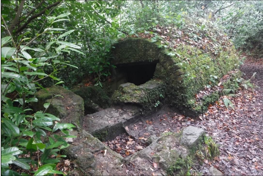
Figure 12.42 The Ice House, as viewed from the south
