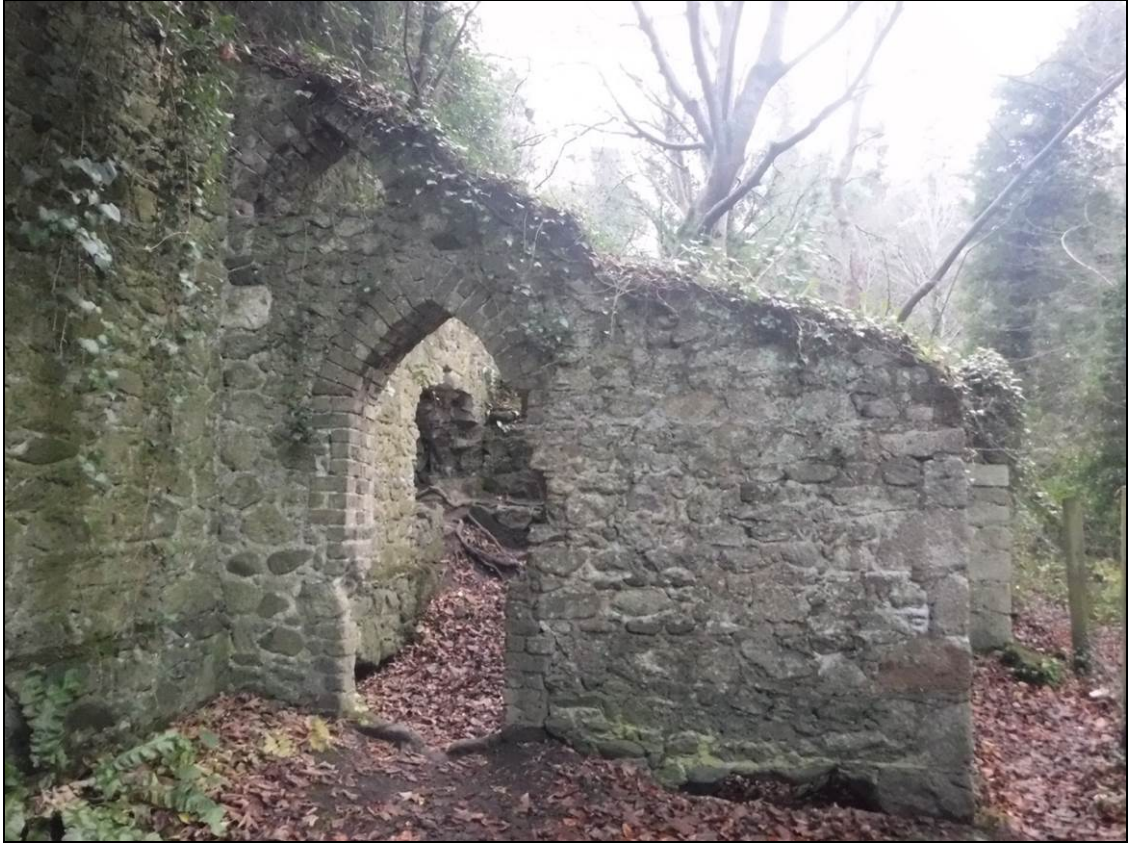
Figure 12.36 The east wall of the boiler house
