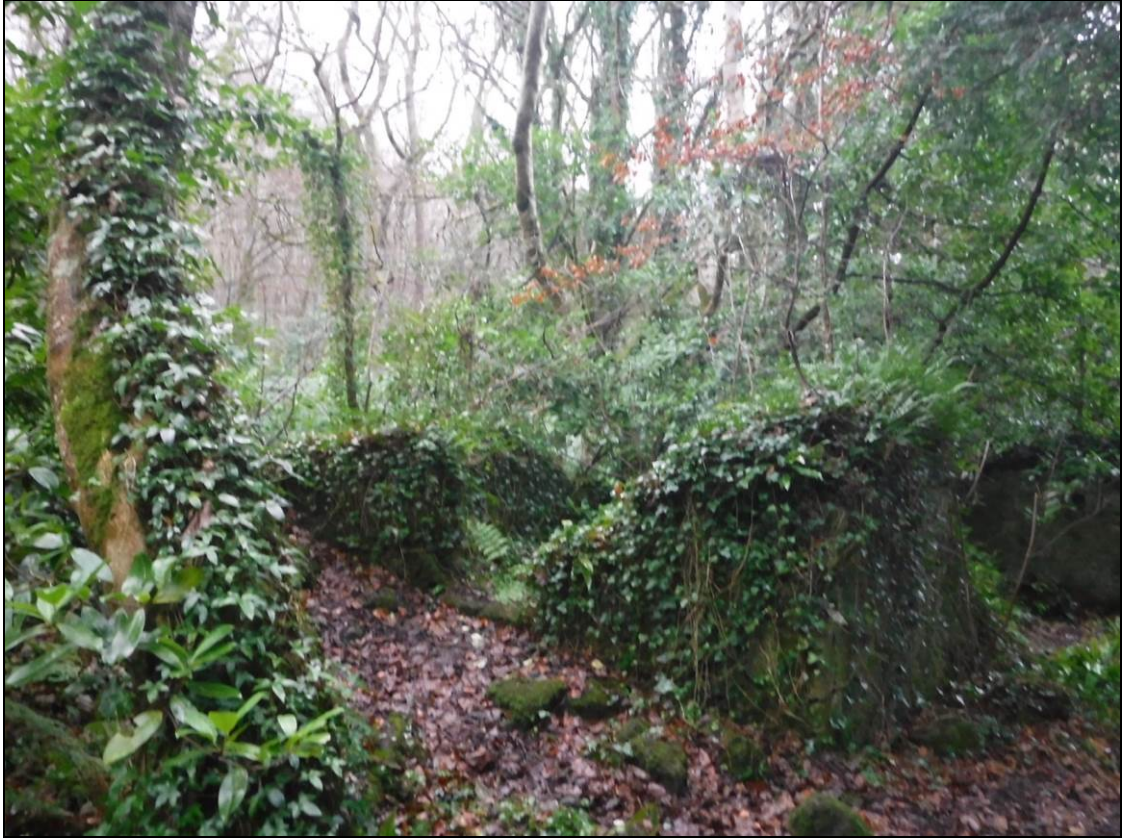
Figure 12.24 Ruined outbuilding in the Kitchen Garden
