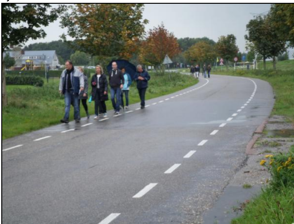
Figure 14.22 Example of a Rural Road in the Netherlands with Advisory Lanes for Pedestrians and Cyclists
