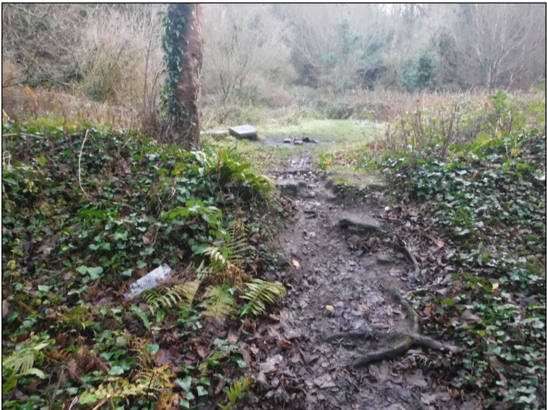
Figure 12.29 The brickwork which is just visible forms part of the foundations of the boiler house which was located within Turner's curvilinear glass house
