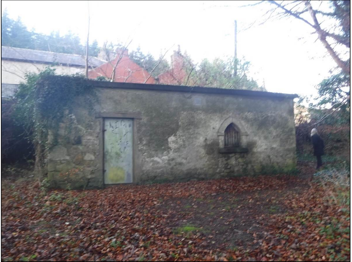
Figure 12.39 East wall of the gate lodge
