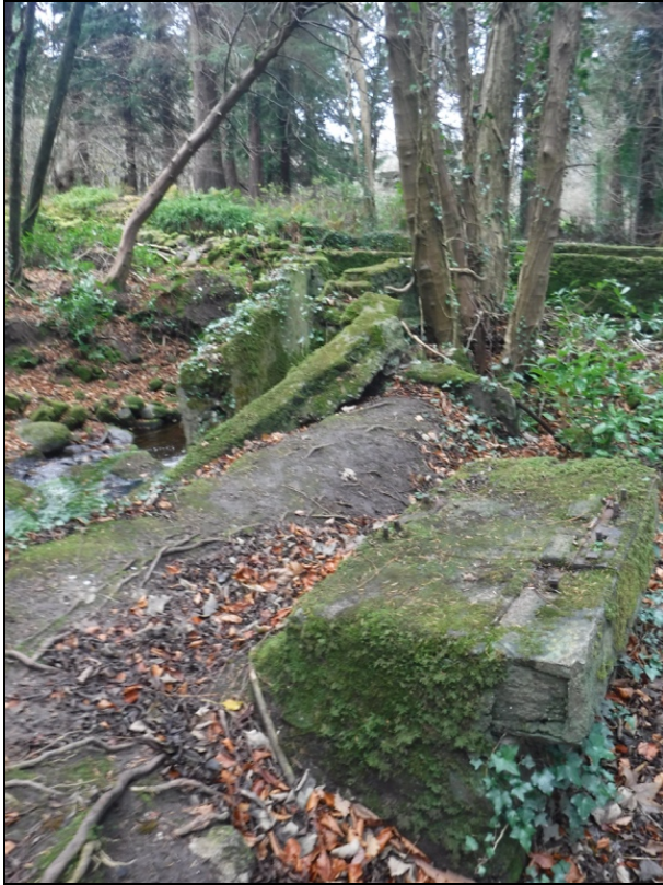
Figure 12.47 The remains of the water wheel, weir and Mill as seen from the south
