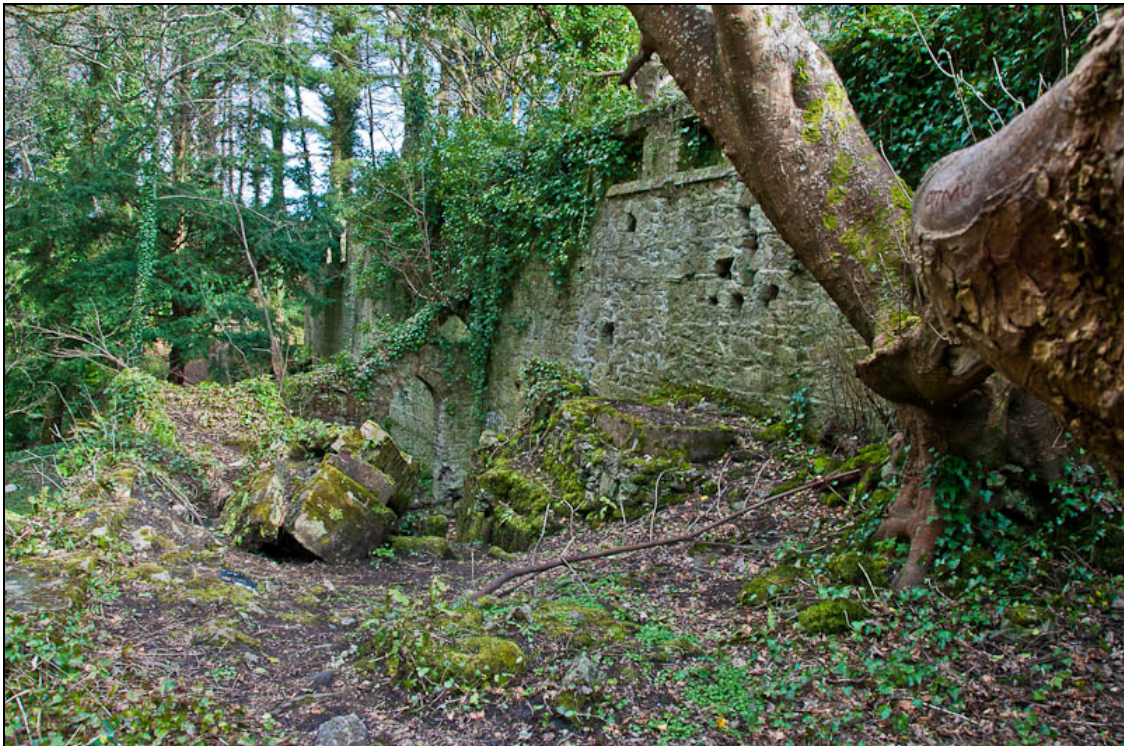
Figure 12.35 The north face of the north wall of the formal garden and the remains of the boiler house
