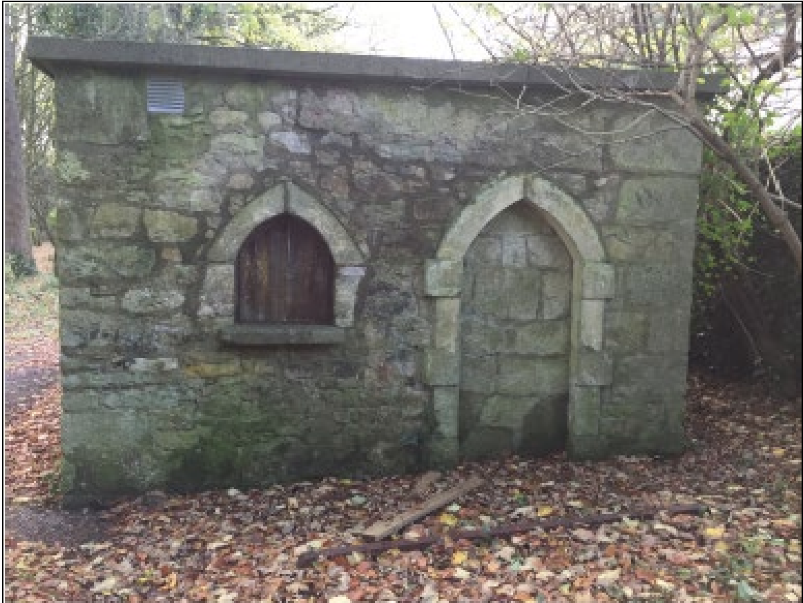
Figure 12.40 North wall of the gate lodge
