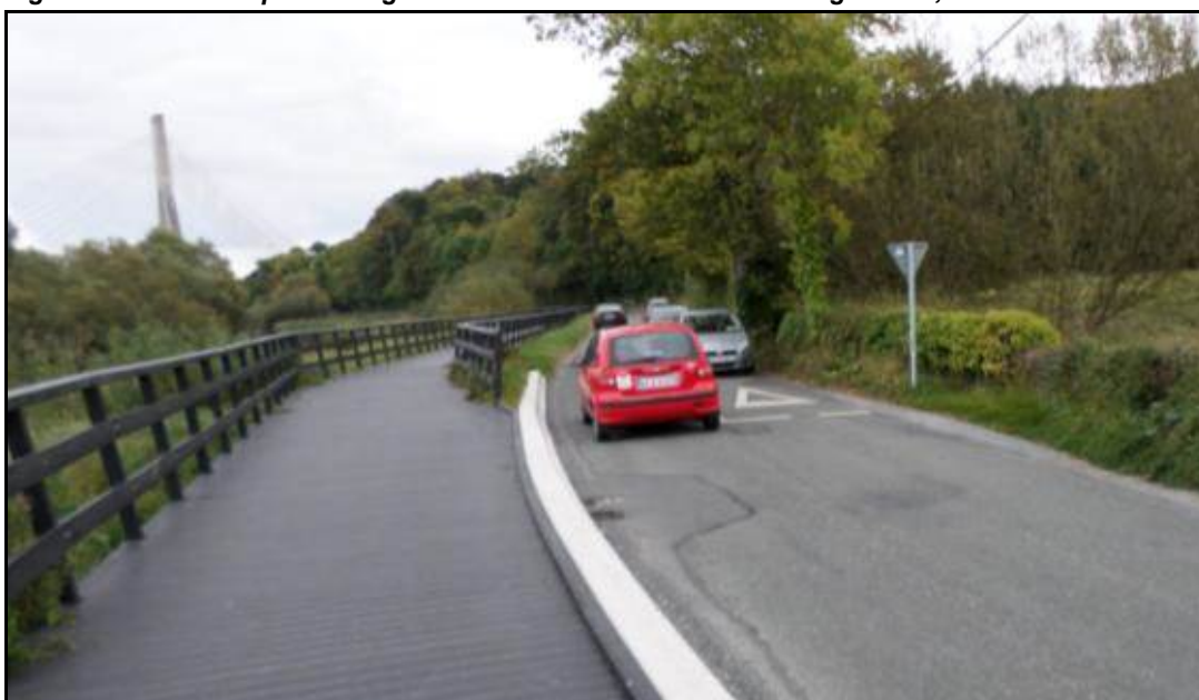
Figure 14.17 Example of Single-Track Traffic Shuttle on Oldbridge Road, Co. Meath
