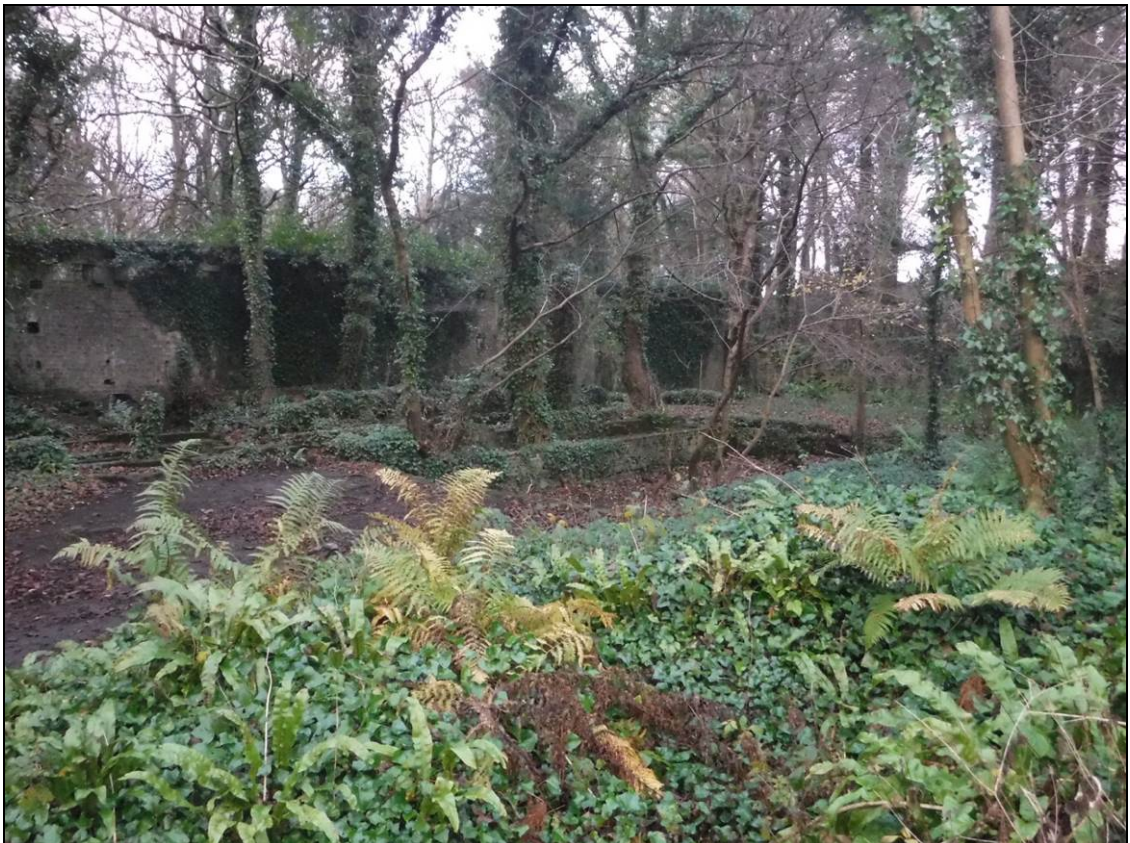
Figure 12.31 Foundations of some of the glass houses with the north and east walls of the walled garden in the background
