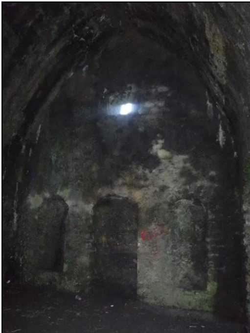
Figure 12.15 The apses in the west wall of the west room on the first floor. The window above relates to the second floor as there would have been a timber floor in between and a vaulted stone roof above.
