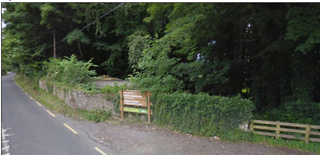
Figure 12.55 The 19 th century boundary wall to Massy's Wood with the gate lodge located just beyond
