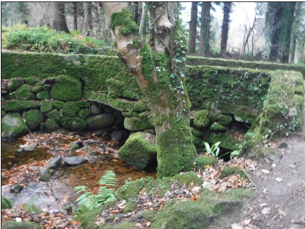
Figure 12.51 Bridge to the north of the Mill Complex
