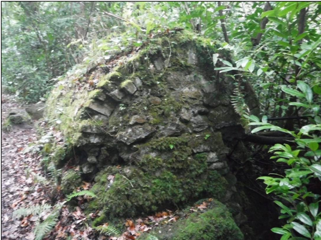
Figure 12.43 The Ice House as viewed from the north
